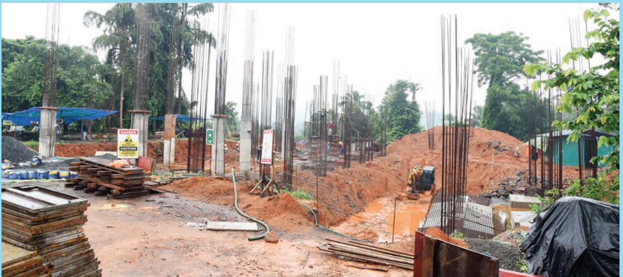
Construction of critical care block at Govt. Medical College, Manjeri
